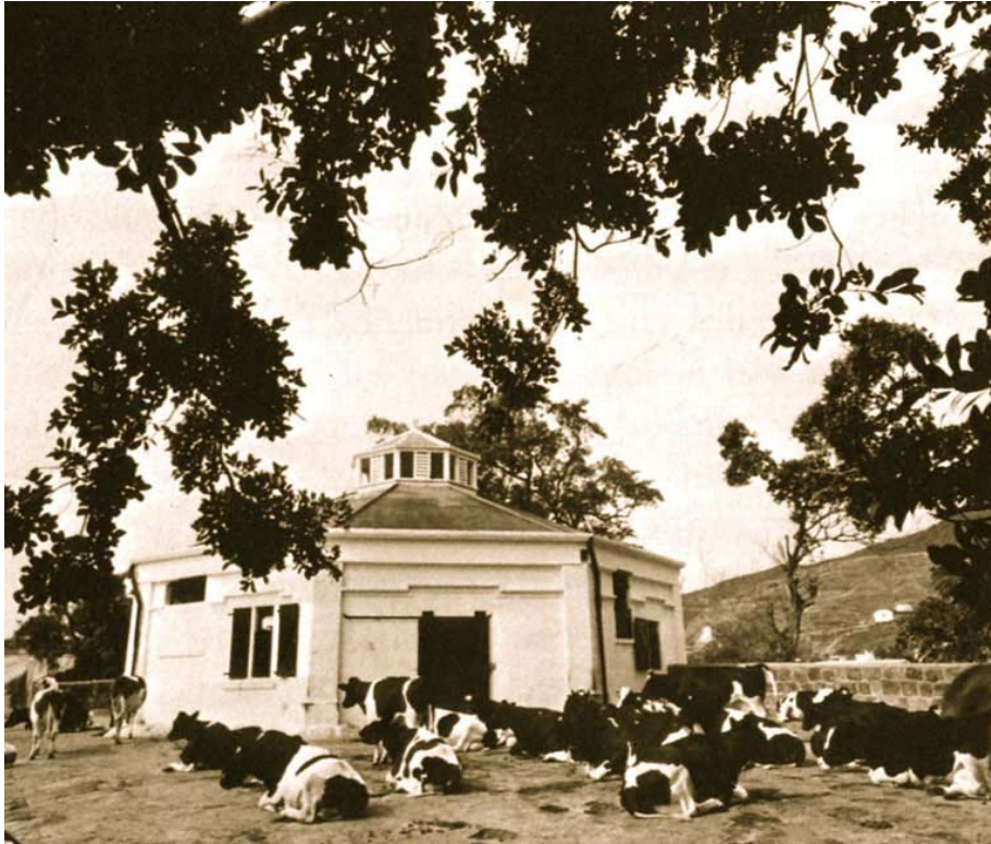
Cowshed before restoration
